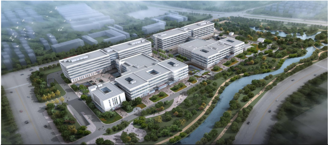
Northern Medical Center Construction
