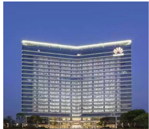
Beijing Huawei Building
